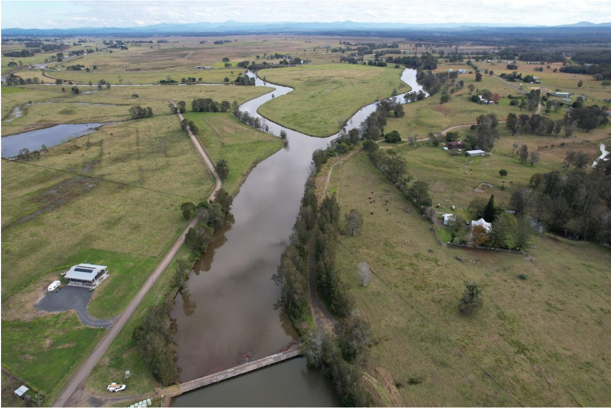
Figure 4-2 The Menarcobrinni floodgates (foreground) and Collombatti-Clybucca floodplain (background) (25 June 2024)
