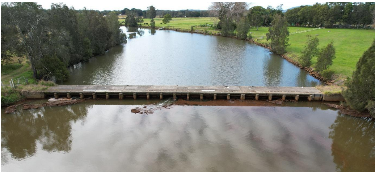
Figure 4-1 The upstream side of the Menarcobrinni floodgates (25 June 2024)
