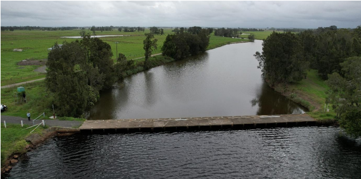
Figure 1-3 The Menarcobrinni floodgates located 3 km downstream of the wetland
